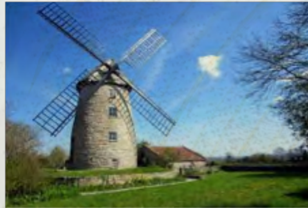
Tower Mills that were built from stone or bricks and had rotating wooden cap that could rotate and take advantage from wind that changes direction.
